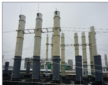
Air Emissions Outlets
