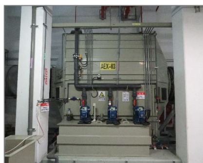
Alkaline Exhaust Gases Treatment System
