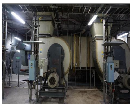
Acidic Exhaust Gases Treatment System
