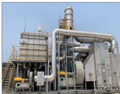
VOC Treatment System
